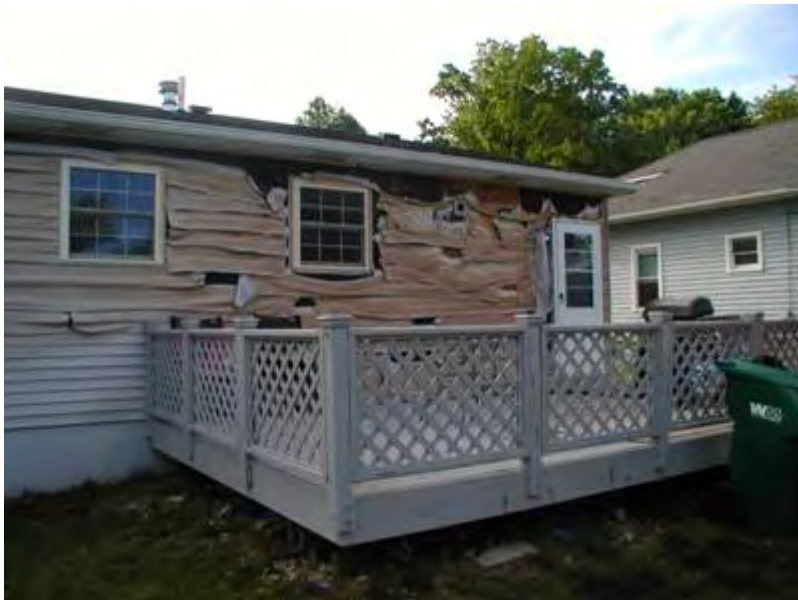
The back side of the house exposed to the fire
